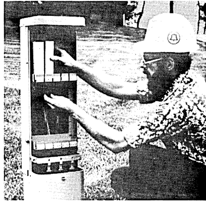
Fig. 19— SLC ™-40 pedestal-mounted repeater enclosure.
