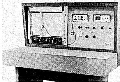
lytical instruments by 5 to 10 times. Its applications include mass spectroscopy, nuclear magnetic resonance studies, and infrared spectroscopy. The system requires no assumptions or computations regarding solutions being sought, and produces results that are not subject to operator interpretation. The self-contained unit sells for about \$15,000. MICRO-TOL ENGINEERING CORP., State College, Penn. For information:
