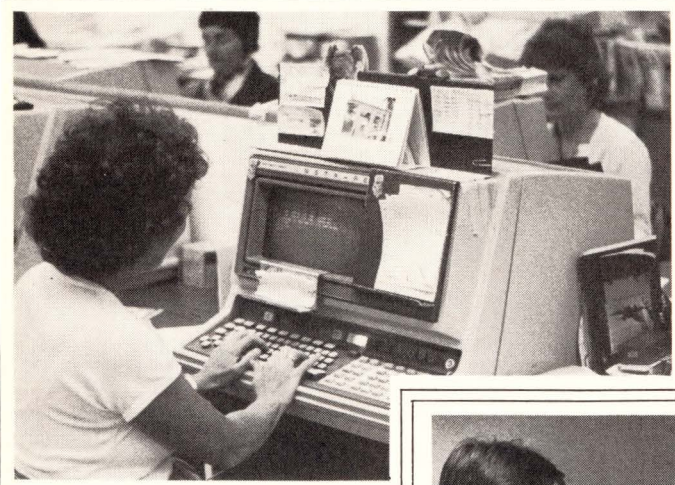
Typical installation where a 125 kW LorTec UPS is powering an Automatic Call Directory (ACD) in an airline's reservations facility.
