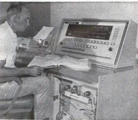
CONTROL CONSOLE at Eleuthera central station directs Mistram site and hand-over to Valkaria. Plotters show missile trajectory and position
