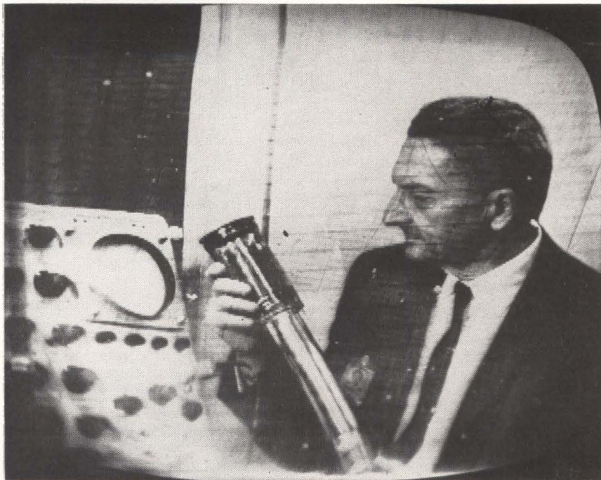
READOUT of a stored picture from tape. Full scan is 0.62 inch high and retrace lines are visible
