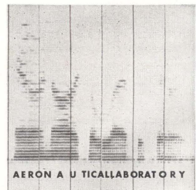
WORDS "aeronautical laboratory" pictorially reproduced by digital computer. Frequency bands are vertical and time is horizontal. Greatest energy is shown by the darker bands
