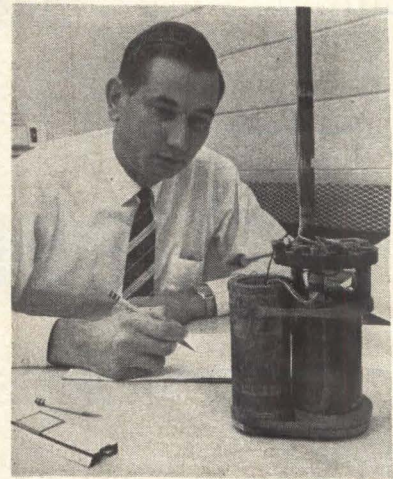
COMPACT 375-joule energy source developed by Ion Physics. A 50-liter coil, including dewar, can store 100 joules, while capacitor banks require 750-liter volume for the same job
