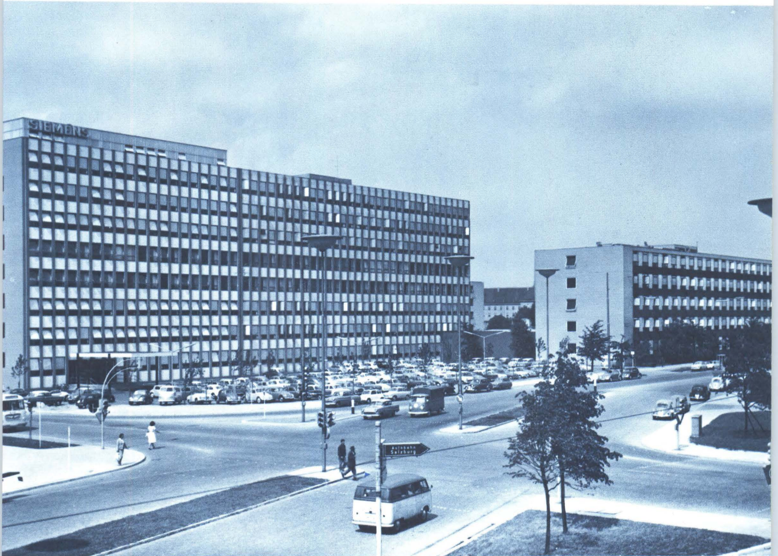
Siemens Components Center, Munich—Main Offices, Research, Manufacturing and Sales
